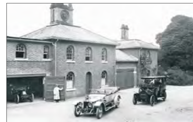
Pell Wall Hall, The Garage 1911
